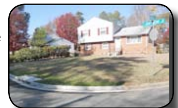
Newly installed catch basins on Larrymore Road in the 9th District
